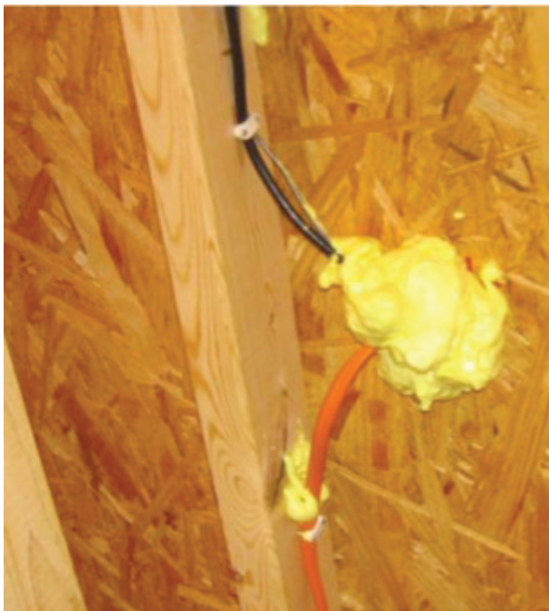
(top left) Taping seams to air-seal a home has been adopted by most FAHE members as well as other groups constructing energy efficient homes. (top right) Duct work run through conditioned space. (bottom left) Spray foam insulation can be used to seal any areas that need to be air-sealed, such as outlets. (bottom right) Fourteen-inch thick walls filled with cellulose insulation.
